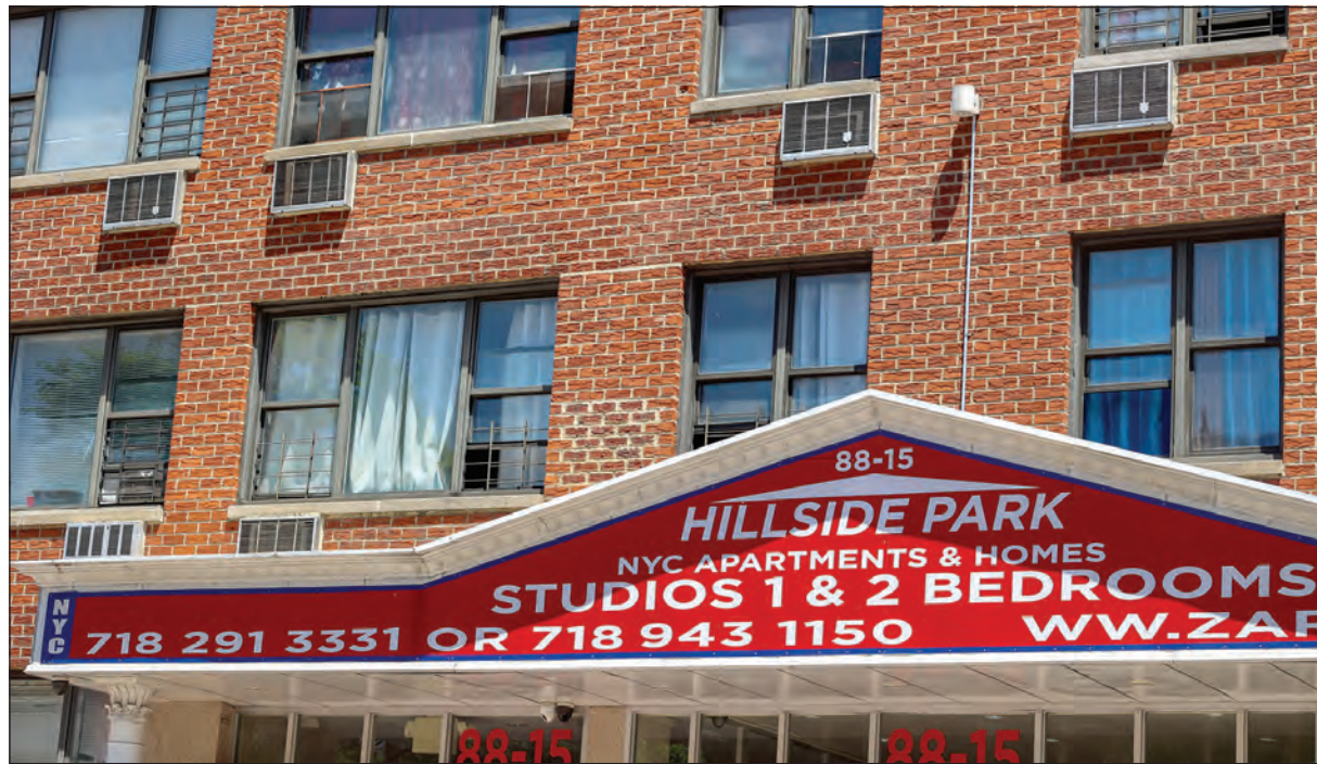
Queens-based Zara Realty has allegedly jacked up rents in many of their local buildings by allegedly inflating improvement construction costs to the state. Eagle photo by Ryan Schwach
