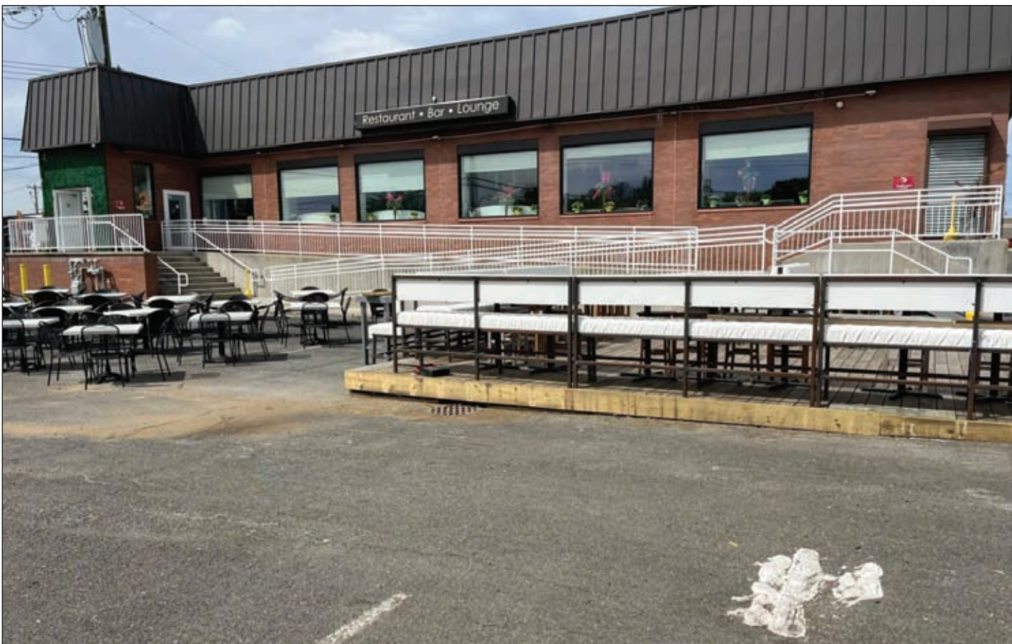
Con Sofrito built a structure on its front lot without permission from the landlord.
