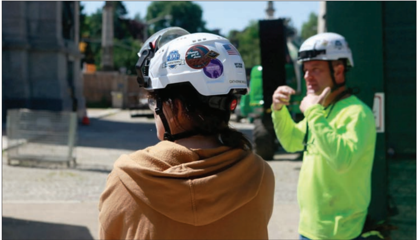
A construction worker at Grand Army Plaza in Brooklyn adorned her helmet with a "Women get it Done" sticker, May 28, 2024.
