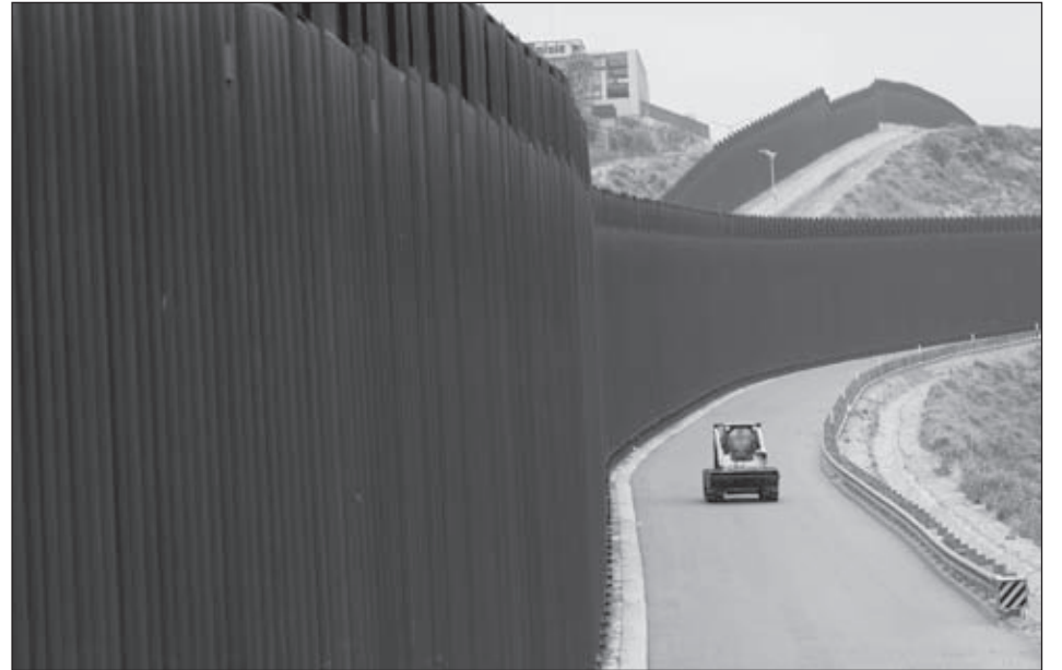
A construction worker drive along the border walls separating Tijuana, Mexico, from the United States, Tuesday, June 4, 2024, in San Diego. President Joe Biden has unveiled plans to enact immediate significant restrictions on migrants seeking asylum at the U.S.-Mexico border as the White House tries to neutralize immigration as a political liability ahead of the November elections.
