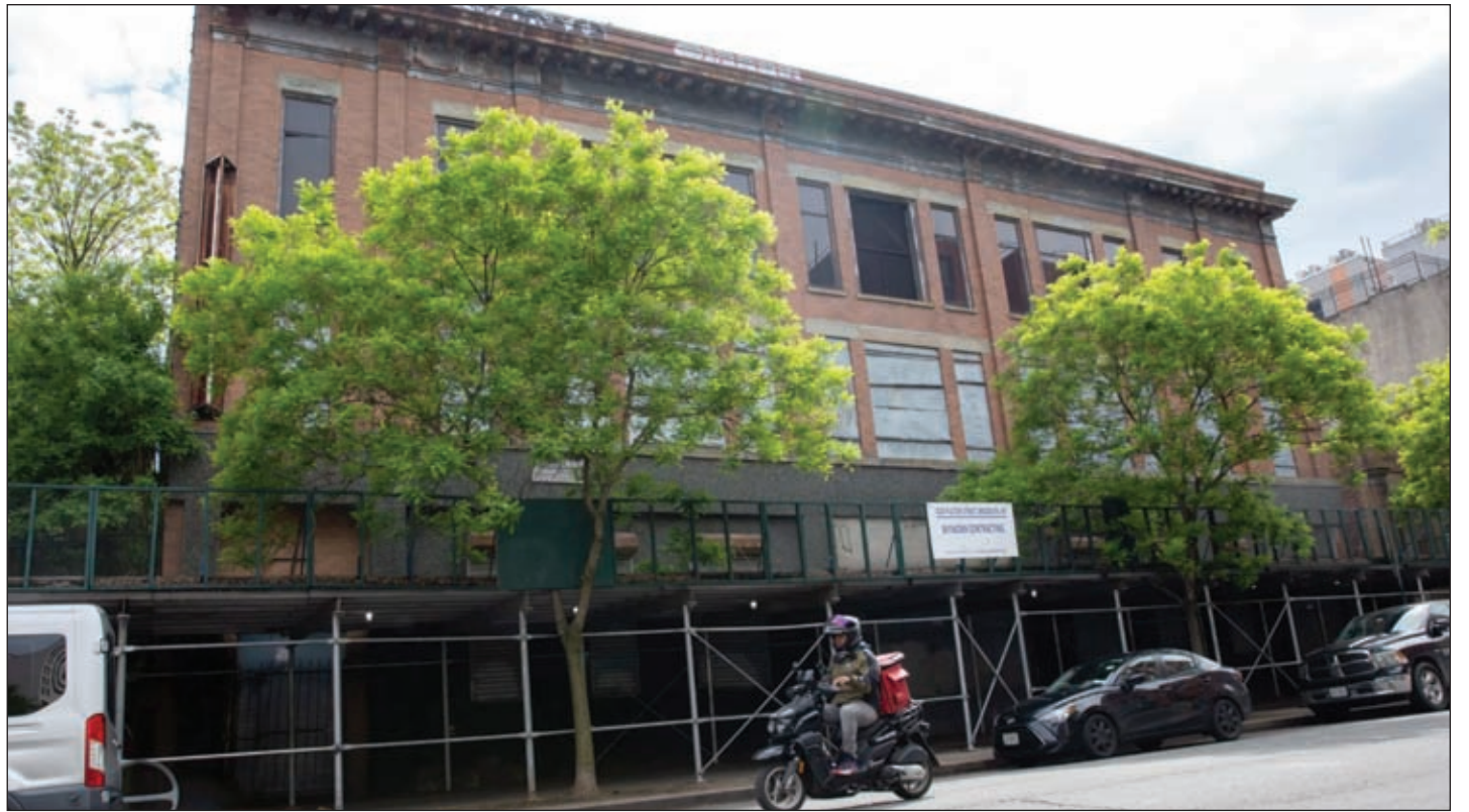
The state is preparing to demolish a derelict building it owns at 1024 Fulton St. in Brooklyn, May 13, 2024. Credit: Ben Fractenberg/THE CITY
