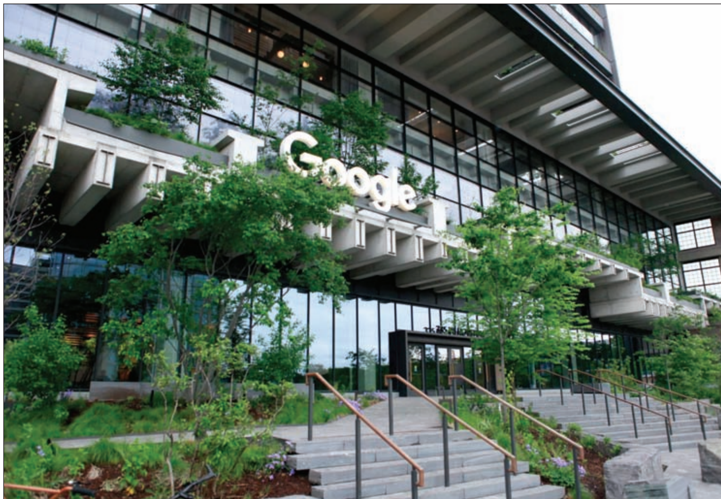
Google purchased office space on the site of the old St. John's Terminal near Hudson River Park in Hudson Square, May 10, 2024.
